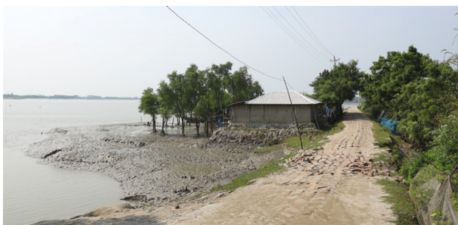
◀ Figure 9: Rural house and roads exposed to the tide in Anulia Union, Assasuni Upazila, Satkhira (IDE, 2022)
