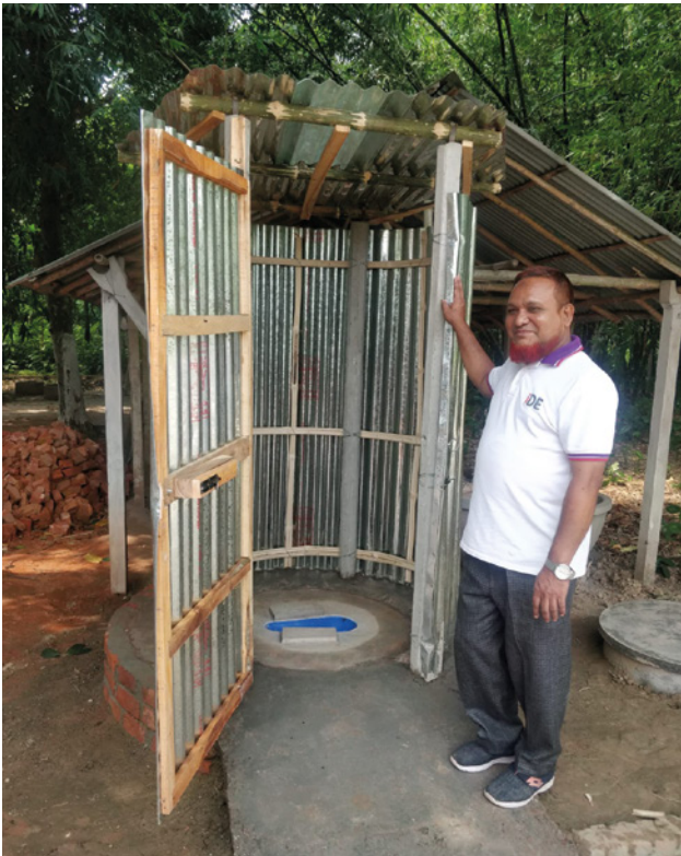
▶ Figure 15: Improved latrine structure with necessary attributes to make it more resistant to floods (raised platform) and to strong winds (circular shape, durable materials). The toilet also has ventilation, lighting and a ramp to enable access by physically challenged people (Md. Nahiduzzaman, 2022)
