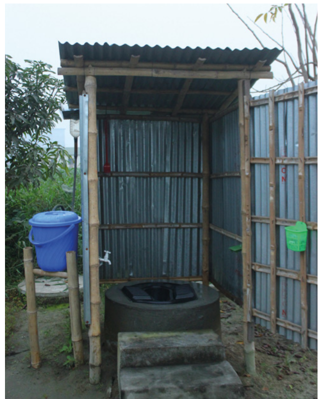
► Figure 14: A latrine superstructure with a handwashing station fed by rainwater (IDE, 2017)
