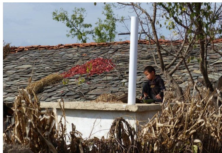
Double pit latrines are currently promoted by SDC as an adapted, safe technology which allows for human wastes to be used as resources.
