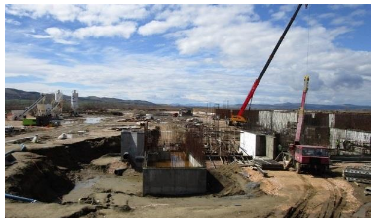
Construction of the wastewater treatment plant Kocani (December 2017)
