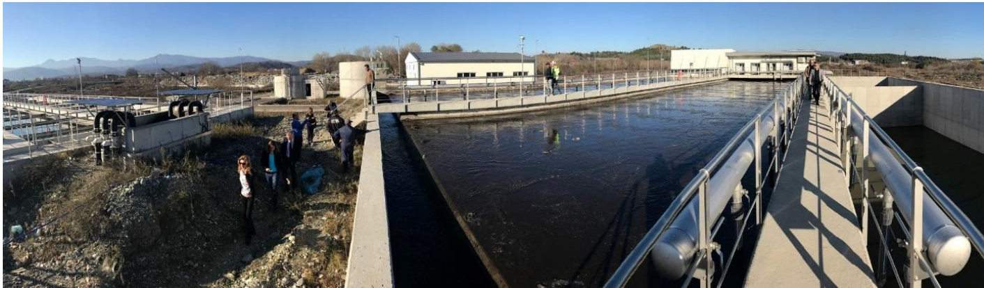
Testing of wastewater treatment plant Gevgelija (January 2018)
