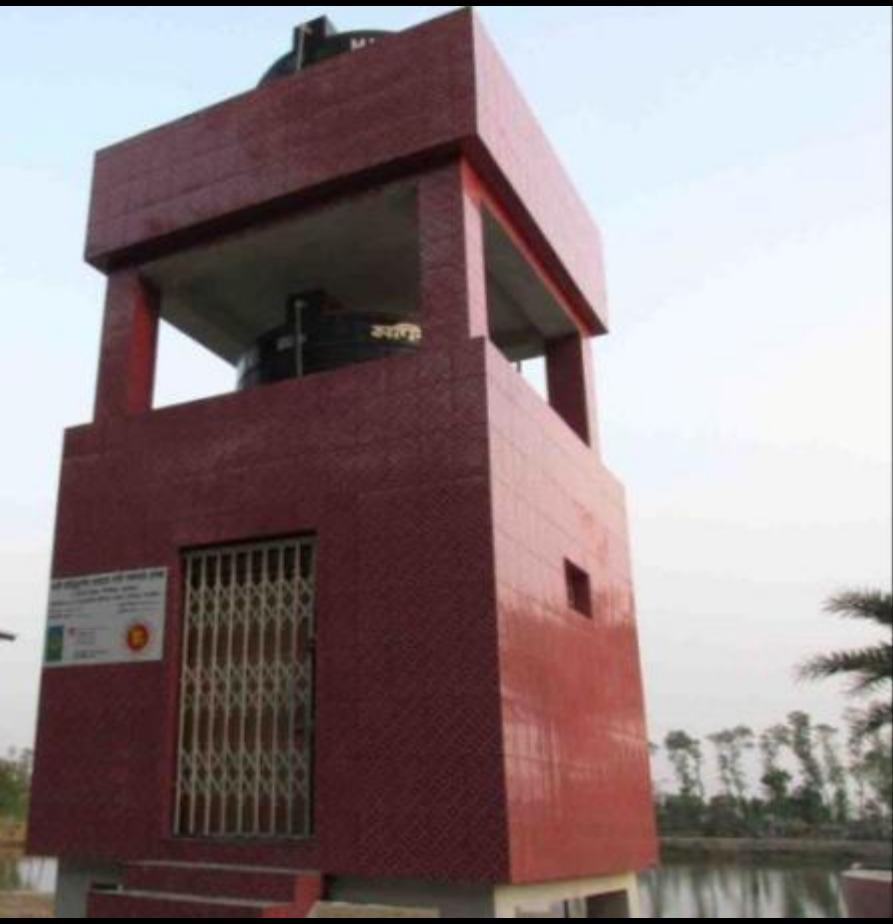
Surface water treatment
