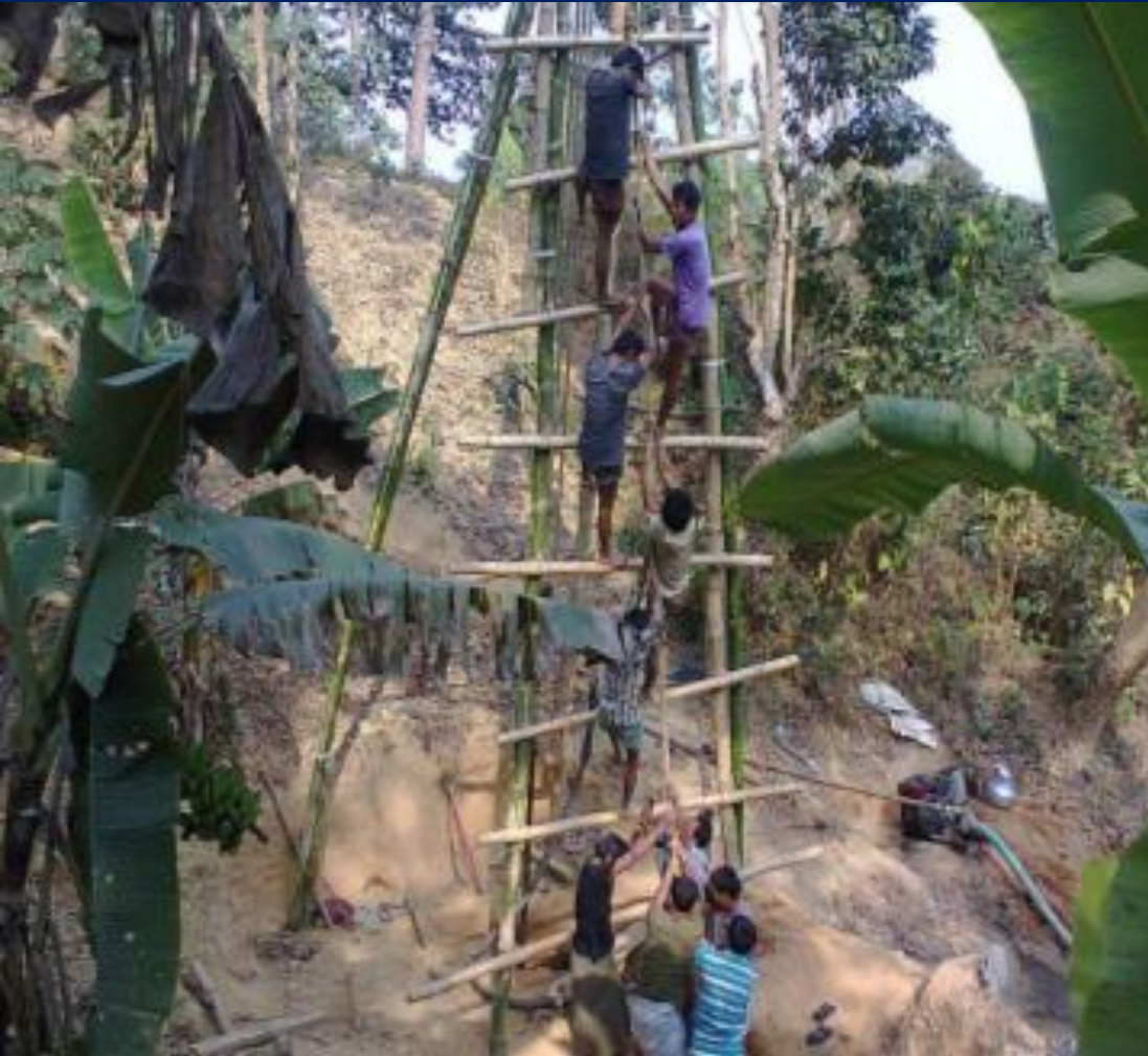
Hand pumps (95%) Depth 250 m
