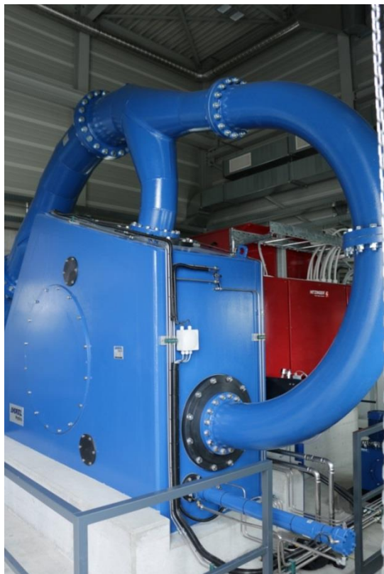
Morgental, St. Gallen, Switzerland 190m, 850 l/s, 1,300 kW
