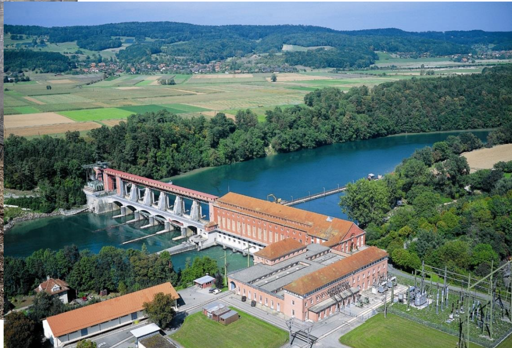
KW Niedergösgen, Switzerland
