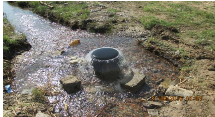
Artesian well after rehabilitation and well development
