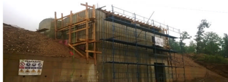
Construction of drinking water reservoir
