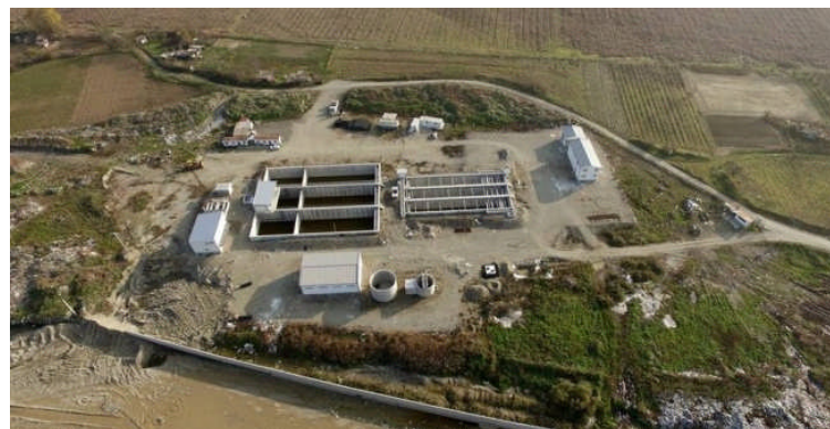
Construction of the WWTP in Gevgelija
