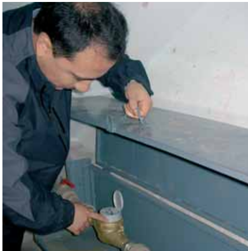
Khujand: Khukand: Water meters are important for equal treatment of users and to encourage payment of bills. (Photo: M. Gysin, SECO)
