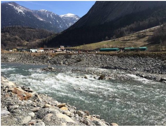
Figure 9. Bloc ramp for fish migration.
