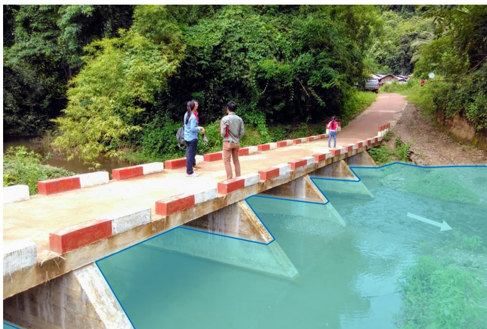
Engineers from the Poverty Reduction Fund (PRF) and SDC Regional DRR Advisors conducting a risk assessment at a newly constructed bridge in Chomphet District, Luang Prabang Province, Northern Lao PDR, 2017 ©SDC, M. Krüger.
