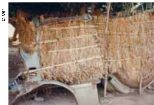
Plate 62 Unusual maize store construction utilizing the shell of an old car
