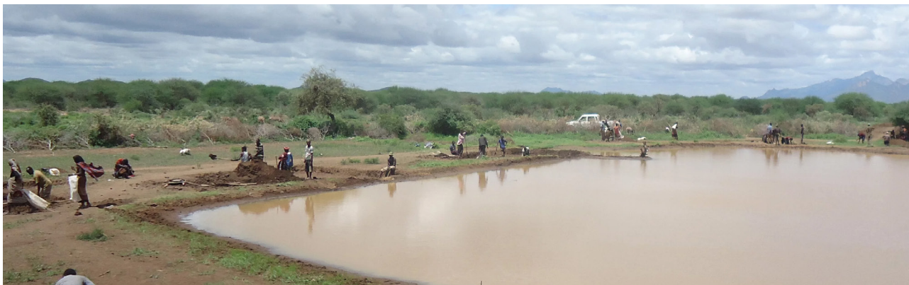
Because of the drought of 2017, rural people in Ethiopia deepen the drenching pond so that more water can be collected.
