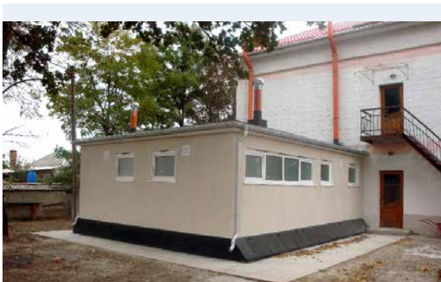
Example of ecosan toilet blocks attached to existing school buildings
