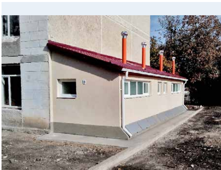
Example of ecosan toilet blocks attached to existing school buildings
