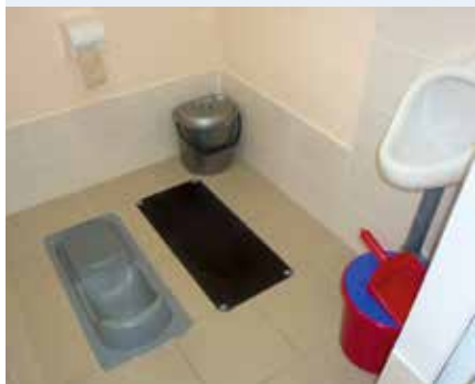
Inside view of an ecosan toilet cabin (squatting type)
