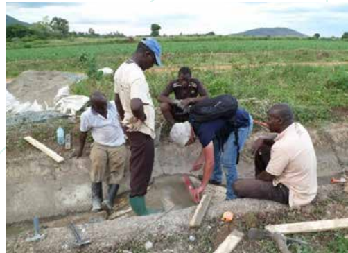
Figure 51: Construction of the weirs in the Main canal
