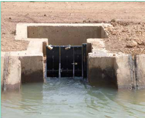
Figure 4: „Modules a masque” for water distribution between the lower level canals
