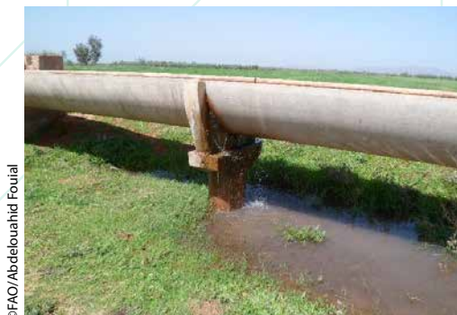
Figure 41: Modules a masques offtakes for flow control
