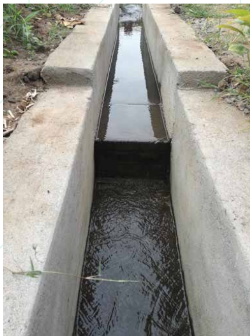
Figure 53: Weirs at tertiary canal level in Division 8
