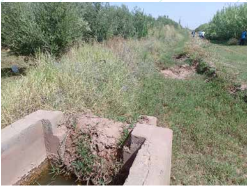
Figure 14: Abandoned quaternary canal filled with sediment
