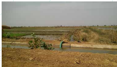
Figure 31: Complete vegetation removal around the lined canals
