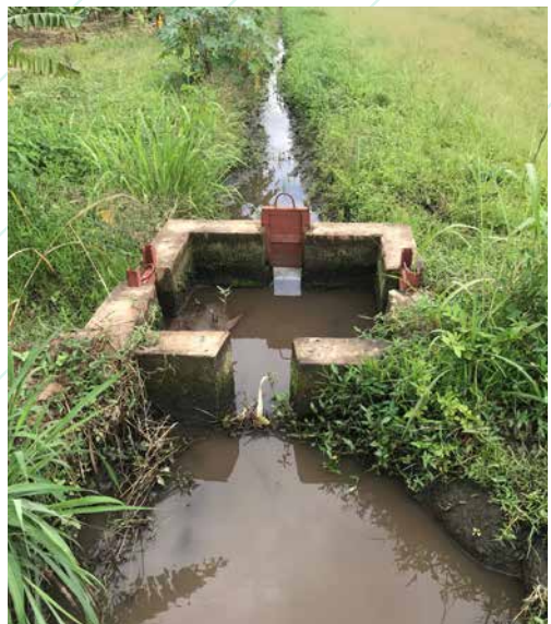
Figure 13: Widened and deteriorated earthen canals
