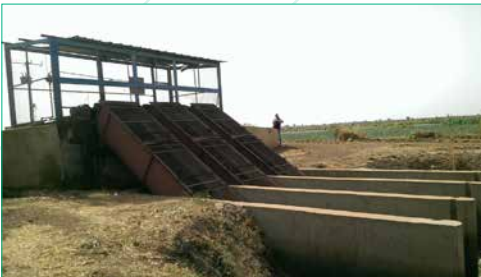
Figure 4: „Modules a masque” for water distribution between the lower level canals
