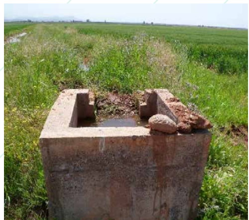
Figure 44: Weed spreads around the hydraulic structures and cover the ditches
