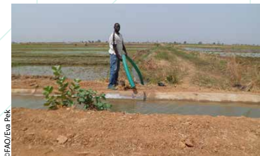
Figure 35: Syphoning from the secondary canal into the rice basins
