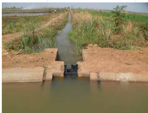
Figure 39: Repaired and reinforced “modules a masques” with concrete chambers
