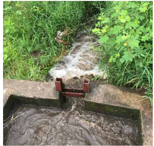
Figure 13: Widened and deteriorated earthen canals
