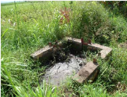
Figure 60: Distribution box and the border of the farm covered by weed
