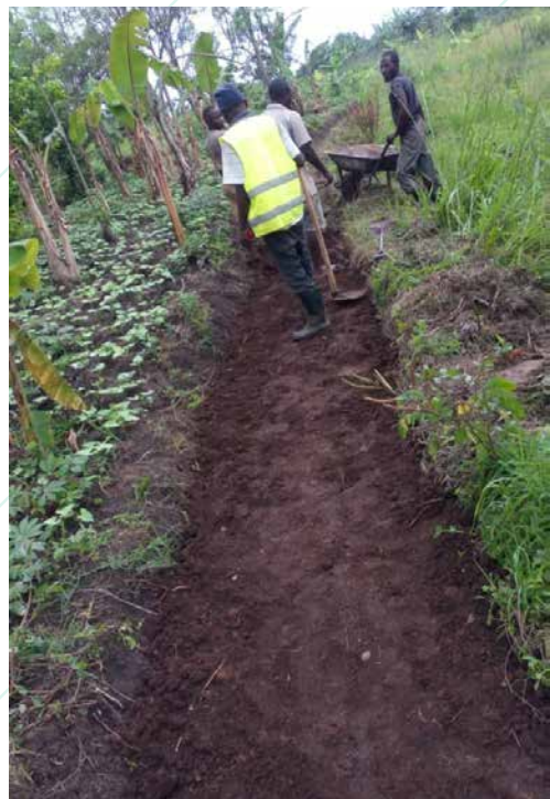
Figure 57: Construction inspection before the lining of quaternary canal
