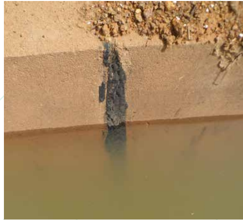
Figure 33: Conditioning the cracks with pitch
