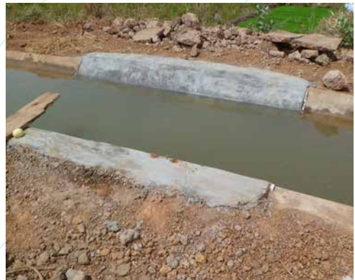
Figure 28: Repaired canal bank with concrete filling and compacted soil
