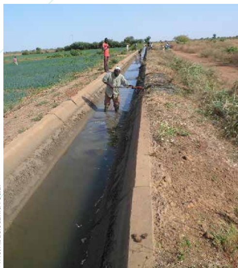
Figure 32: Enlarging cracks in the secondary canal
