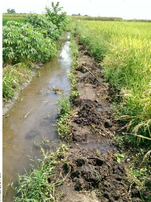
Figure 50: Sedimentation deposit in quaternary canals
