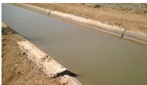
Figure 32: Enlarging cracks in the secondary canal
