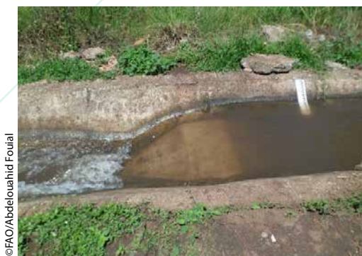
Figure 75: Gauge station at the weir in the secondary canal
