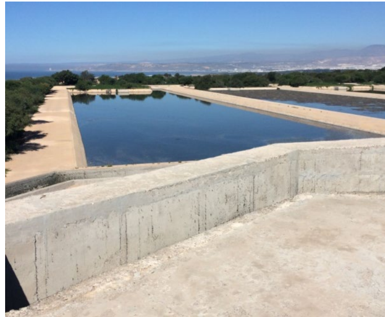
The wastewater treatment plant M'zar in Agadir
