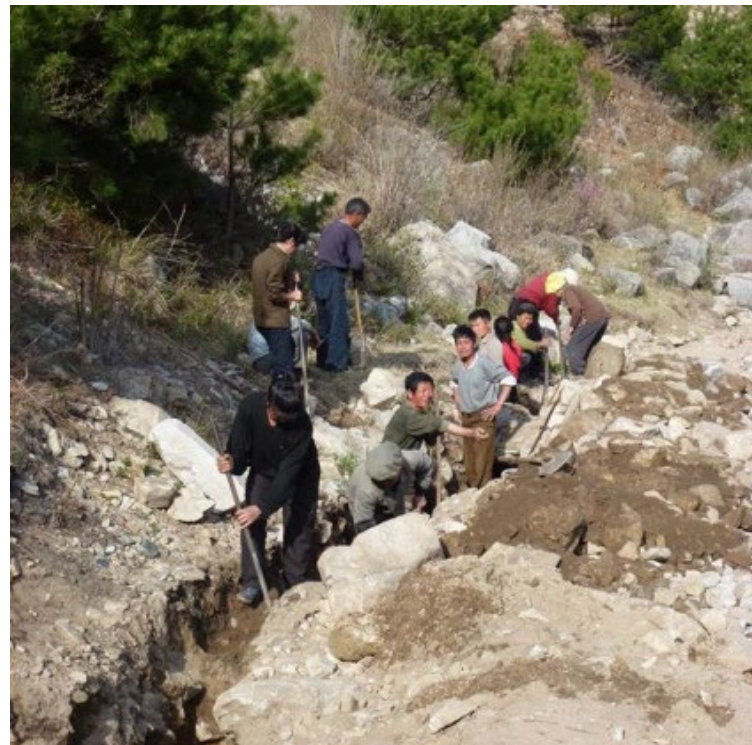
Locals building WASH infrastructure in remote areas in DPRK
