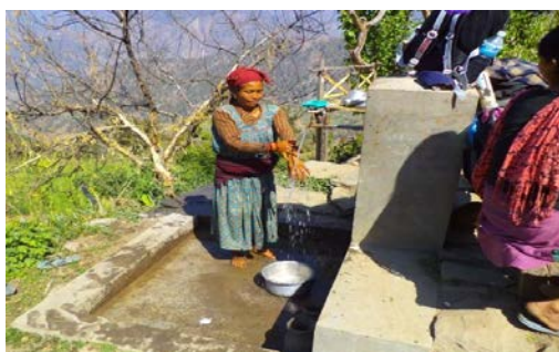
Photo 5 WTCT cleaning tapstand, Jajarkot
