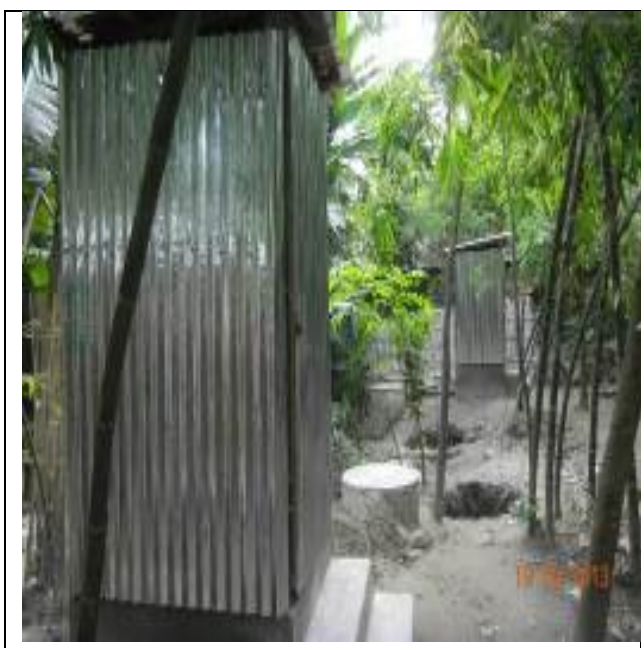
Picture: 6 Latrine support from Tdh
