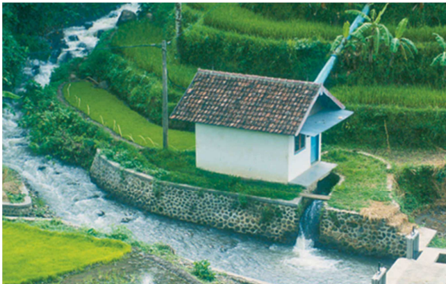
Small hydropower plants like this one in Indonesia supply rural areas with sustainable energy.
